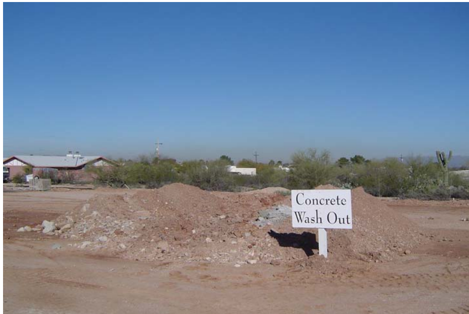
Designated concrete wash out area
