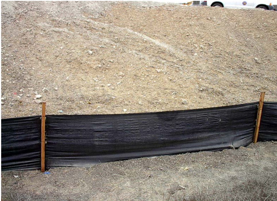
Silt Fence - Good
