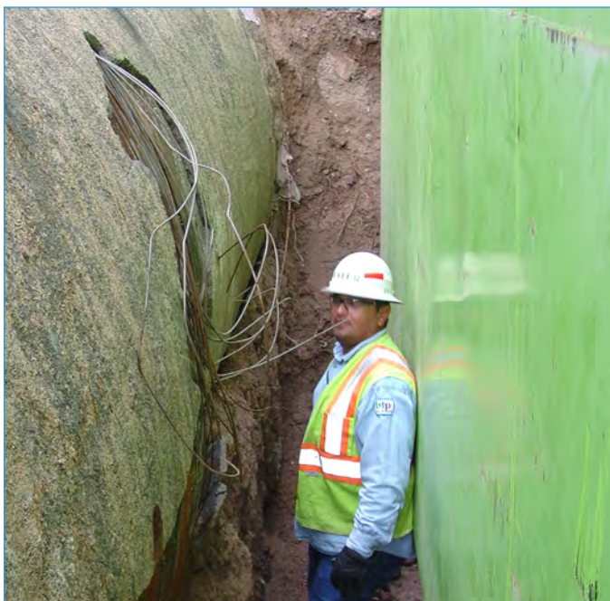
By monitoring its infrastructure regularly, Tucson Water was able to repair a 96-inch transmission main from the Clearwell Reservoir that was at risk of failure.
